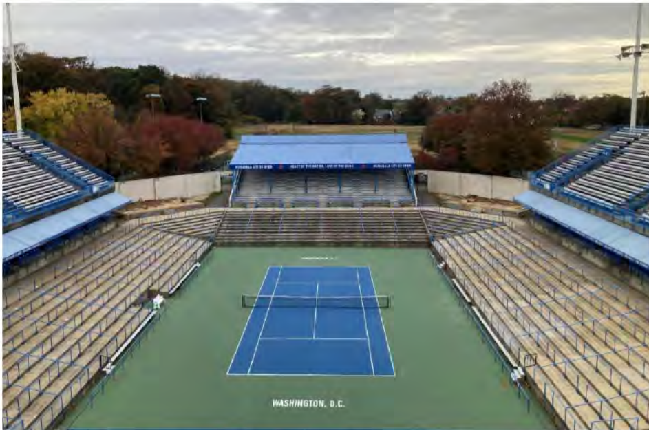
Aerial View looking North from the stadium at the Rock Creek Tennis Center (Source: NPS File Photo)
