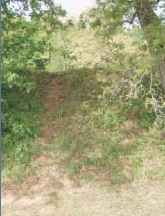
Visitors damage Star Fort's earthen fortifications by climbing on them and causing erosion.
