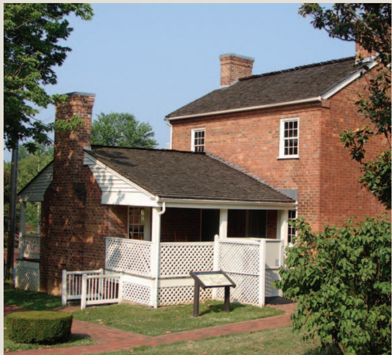
Maintaining historic structures such as Johnson's Early Home is an important responsibility of park staff.
