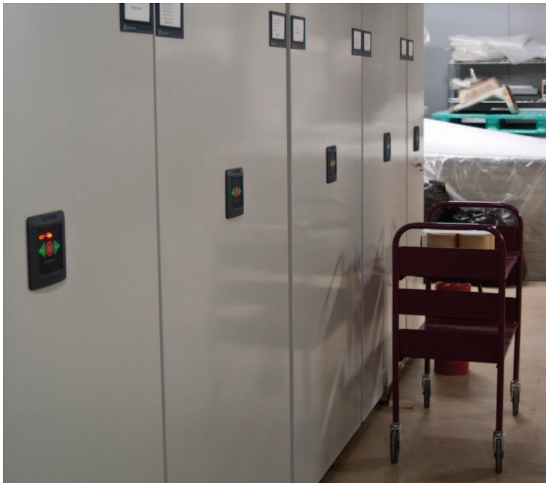
The park has a state-of-the-art Museum Preservation Center that features compact shelving to maximize available storage space.
