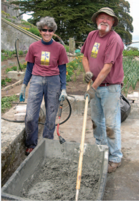
Volunteers from The Garden Conservancy mix cement to restore a raised planting bed in the historic gardens.
