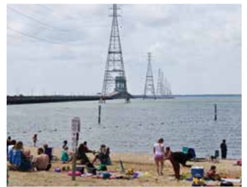
Above: Spring clouds reflected in James River, Colonial National Historical Park, site of first English settlement, Jamestown Island, Virginia. ©Tom Till Right: Seventeen electric transmission towers even taller than these in Newport News, Virginia would forever mar the John Smith Trail and the historic character of Colonial National Historical Park if Dominion moves forward with its ill-conceived proposal. © Margaret Fowler/Save the James Alliance
