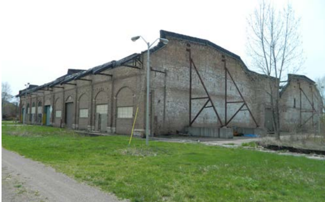
REAR ERECTING SHOPS (NORTH+EAST FACADES)
