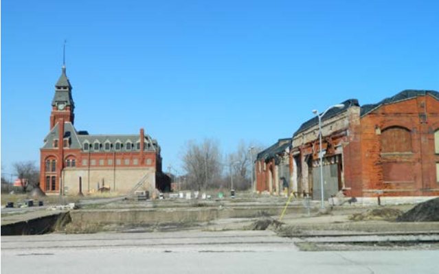
TRANSFER PIT CORRIDOR
