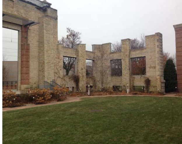
CARNEGIE LIBRARY, SHEBOYGAN, WI
