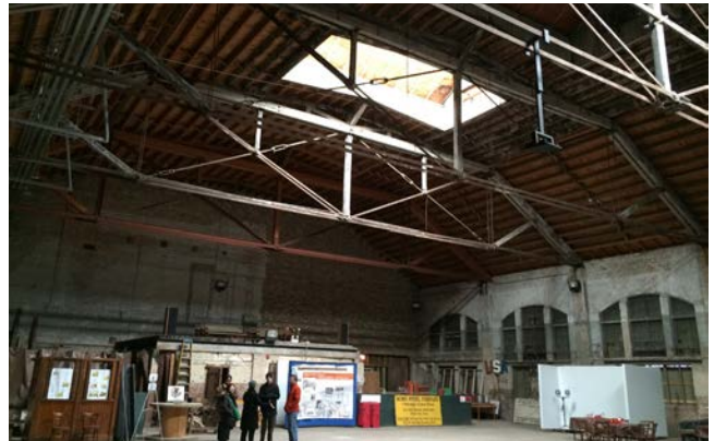
NORTH WING INTERIOR
