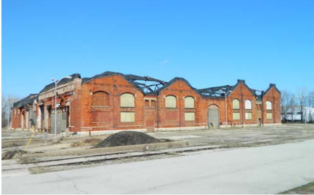
REAR ERECTING SHOPS (SOUTH+WEST FACADES)
