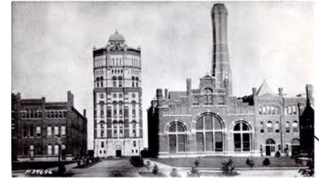
Water Tower, Powerhouse and Iron Machine Shop
