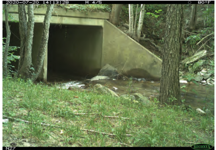
Cold Springs Culvert. Photo: Wildlands Network / NPCA
