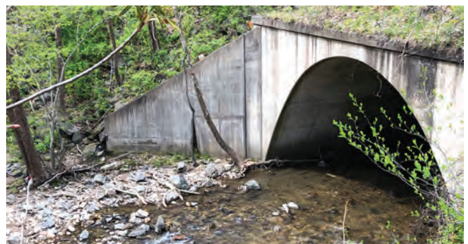
Fines Creek Culvert. Photo: Wildlands Network
