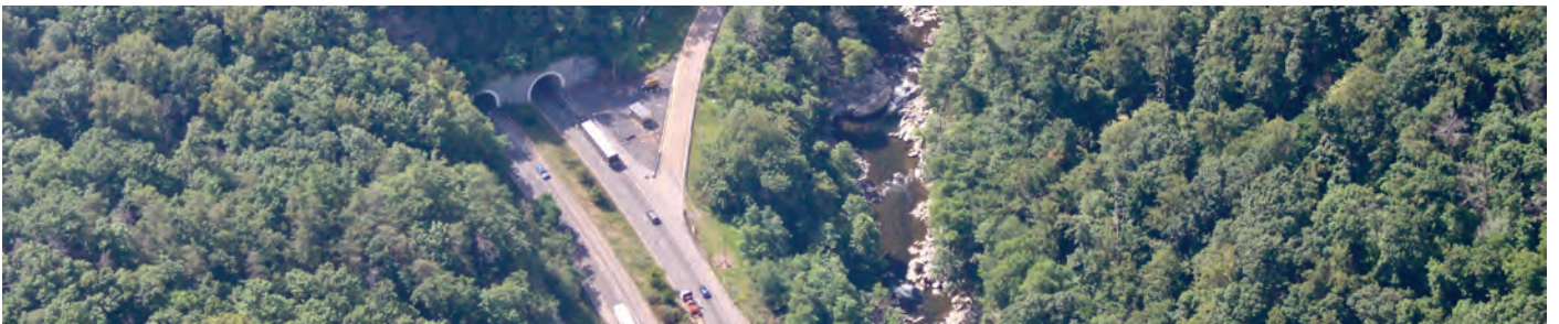
Double Tunnel. Photo: Paul Noah, NPCA and SouthWings
