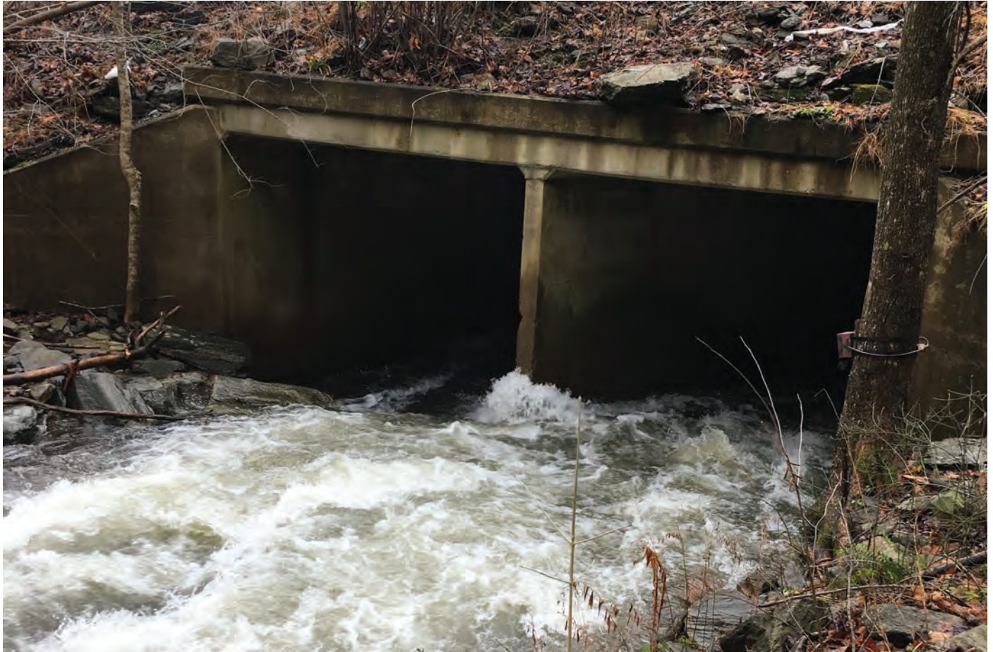
Cold Springs Creek Culvert. Photo: NPCA
