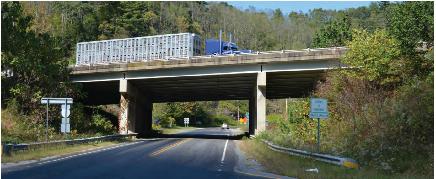
Fines Creek Bridge. Photo: Ron Sutherland
