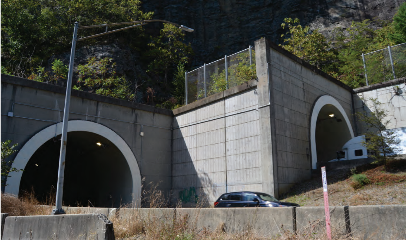
I-40 traffic moves through the Double Tunnel. Photo: Ron Sutherland
