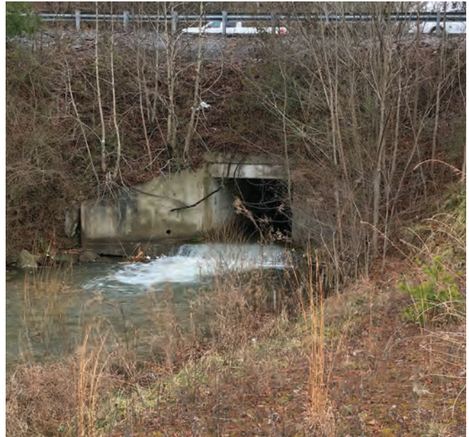
Millcreek A Box Culvert. Photo: NPCA
