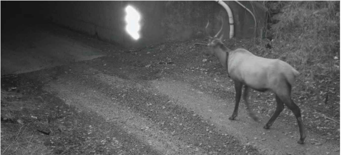
An elk uses Wilkins Creek Box Culvert A to cross under the interstate. Photo: Wildlands Network / NPCA
