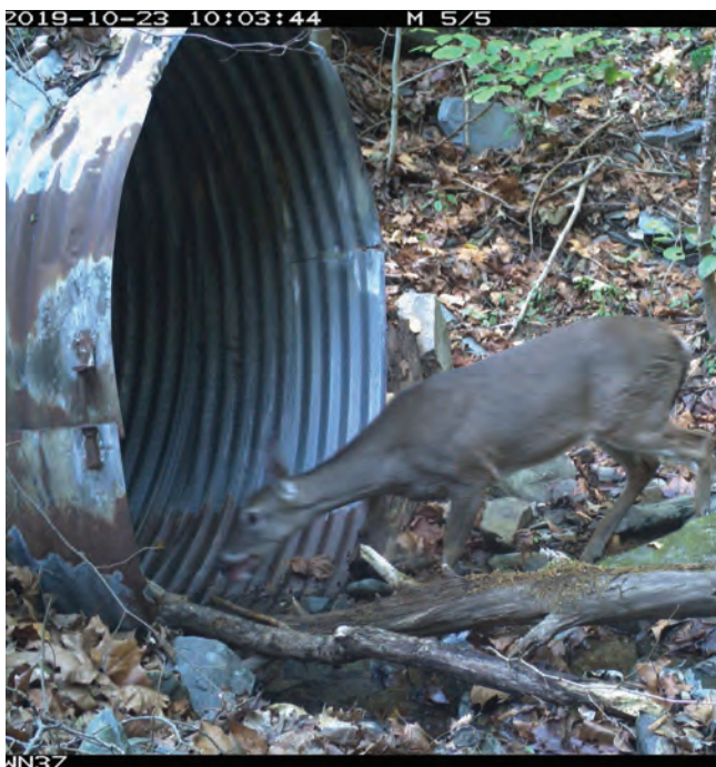
White-tailed deer inspects the Naillon Branch Culvert. Photo: Wildlands Network / NPCA
