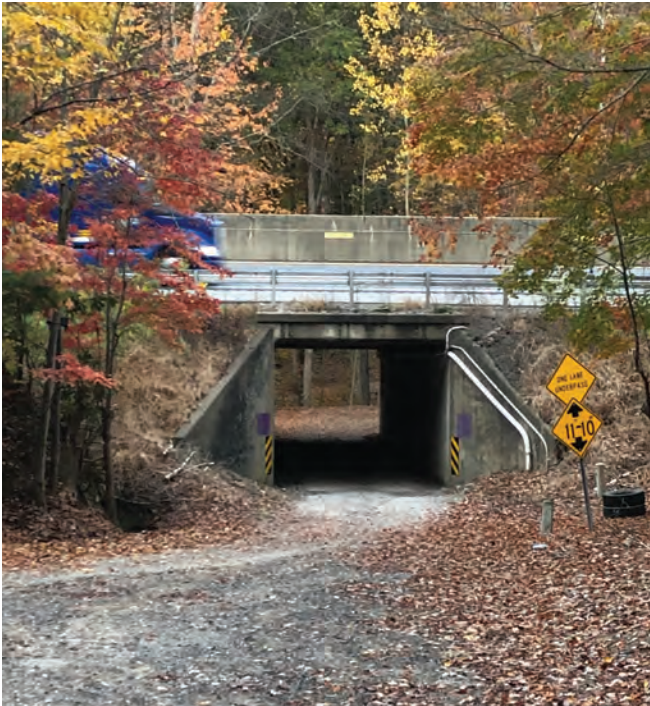
Wilkin's Creek Box Culvert A. Photo: NPCA
