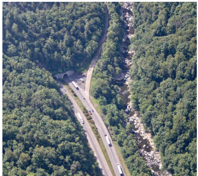
Double Tunnel. Photo: Paul Noah, NPCA and SouthWings
