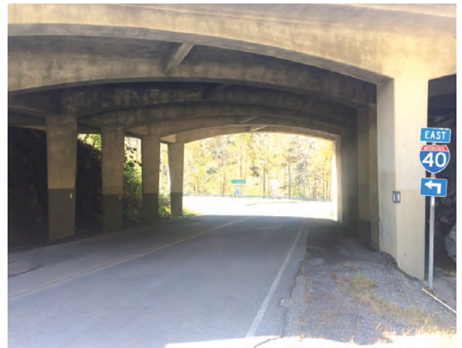
Waterville Bridge. Photo: Wildlands Network
