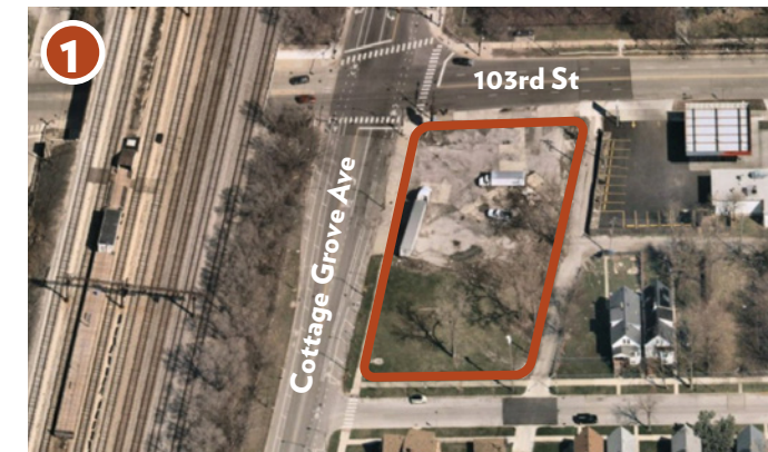
Existing Conditions of POP! Opportunity Site
